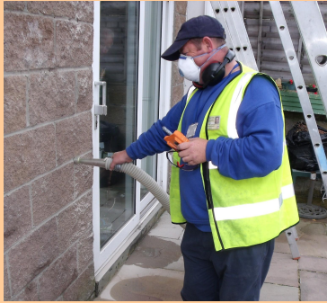
Cavity wall insulation being carried out in St Brelade.
