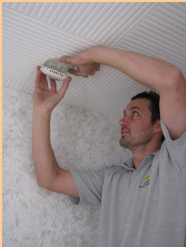
An Energy Efficiency Service contractor installs a new smoke alarm.
